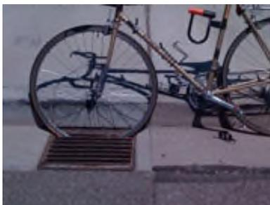
It is recommended that non-complying grates be replaced with bicycle-safe-hydraulically efficient versions. A temporary correction would be to weld steel cross straps or bars perpendicular to the parallel bars at 100 - mm (4-inch) center-to-center maximum spacing to provide a maximum safe opening between straps.
