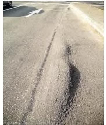
The AASHTO bike guide provides guidance on appropriate bikeway surfaces, including smoothness, drop-offs, depressions and/or irregularities, and locations and types of utility covers and drainage grates. For rideability on new construction, the finished surface of bikeways should not vary more than 6 mm (1/4") from the lower edge of a 2.4 m (8') long straight edge when laid on the surface in any direction.
