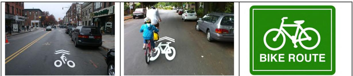
Provides for shared use with pedestrian or motor vehicle traffic. This type of bikeway is commonly found in residential neighborhoods and/or streets with low speed limits. Bike routes may have a wide travel lane and are established by placing "Bike Route" signs along the roadway (MUTCD sign D11-1). They may or may not have shared lane markings ("sharrows") stenciled on the roadway.
