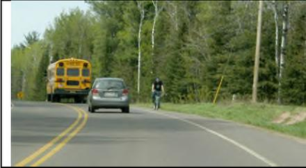
Caltrans points out that it may be inappropriate to designate a rural highway as a bikeway due to limited use and/or lack of continuity with other bikeways. However, they recommend development and maintenance of a 4-foot paved shoulder with a standard 4-inch edge line to significantly improve safety and convenience.
